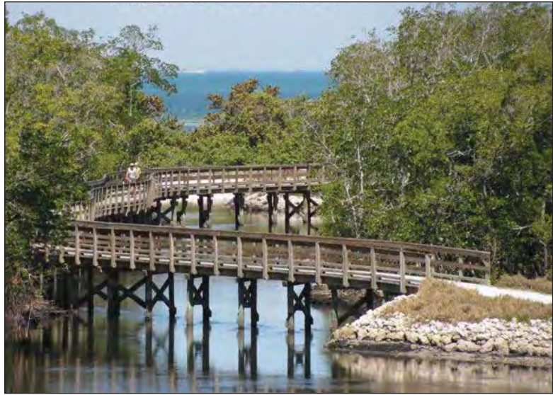
Figure 18-7B. Existing boardwalk in Robinson Preserve.
