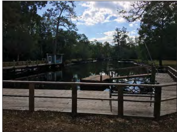
Figure 12-1B. Existing boat ramp and dock facility.
