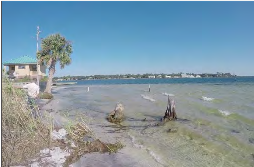
Figure 3-5B. Photograph of eroded shoreline on the east side of Veterans Park.
