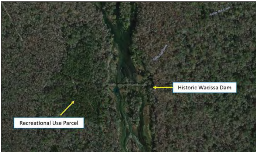
Figure 9-3B. Aerial photograph of the Wacissa Dam site.
