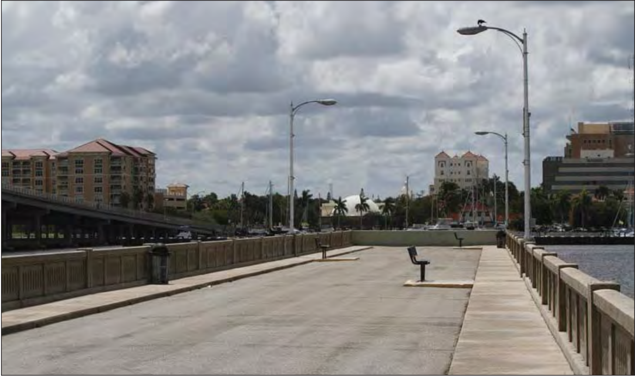
Figure 18-5C. Ground level photograph of the existing concrete fishing pier.
