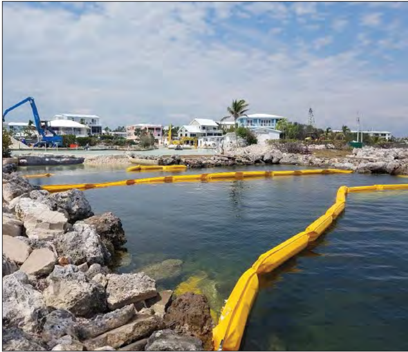
Figure 23-1C. Canal shallowing under construction in Canal #75, Key Largo, Florida.
