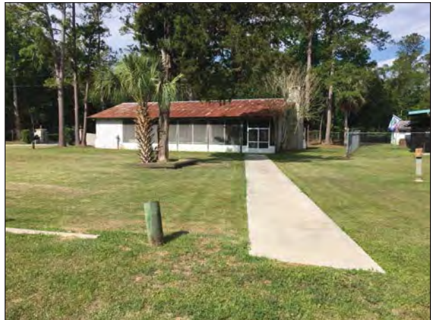
Figure 12-1C. Existing property manager's facility.
