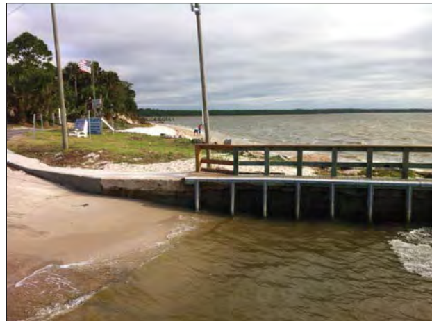
Figure 6-3B. The existing Indian Pass boat ramp.
